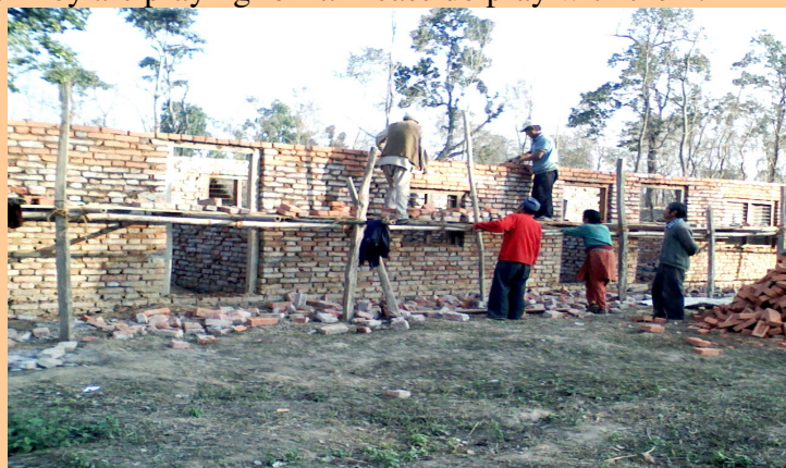
New strong building is being built but need the roof!
