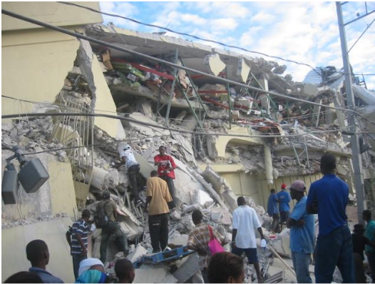
Earthquake impact, January 12, 2010
