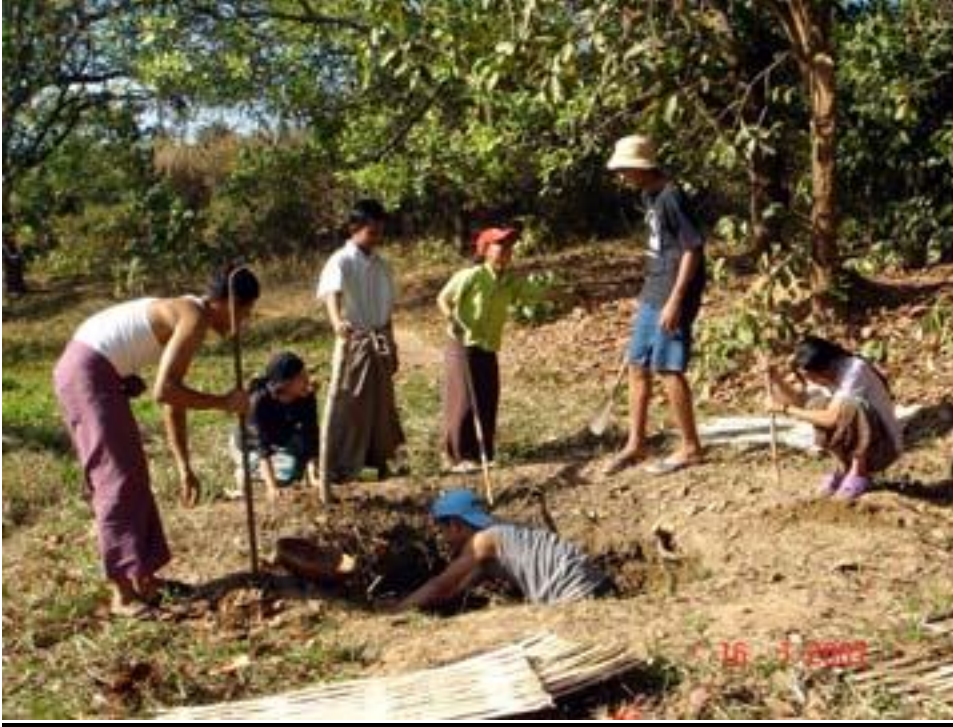
Seed Project (Water Well Repair in Surrounding Community)
